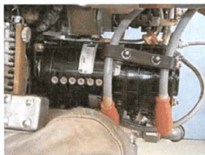
Picture 3: original APU Starter electrical connectors.
